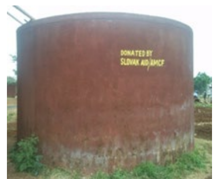
Water reservoir constructed at Naura Secondary School
