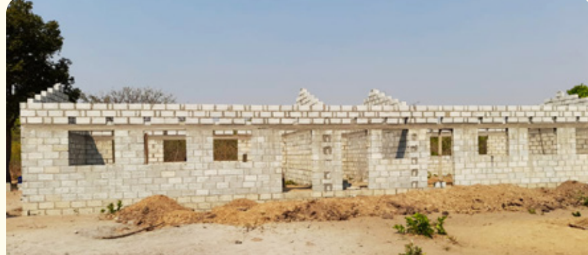
Primary School building near completion
